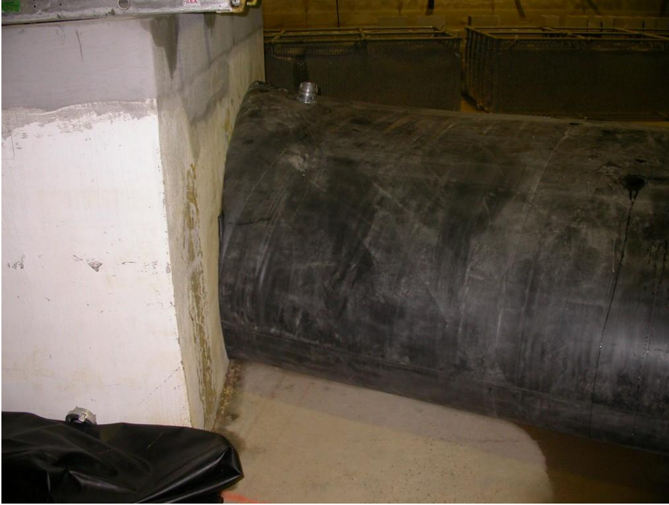
Figure 4. Unit A abutting the wingwall and showing one of the upper fill ports
